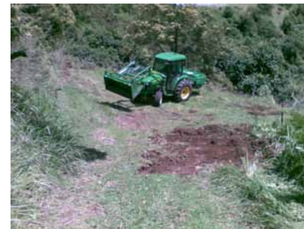
Second switchback widening at 3km Photos: John Harriott
