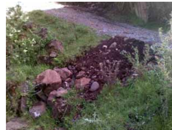
Access road upgrade: First switchback remedied
